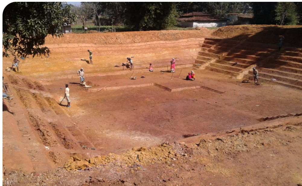
The nearly-completed water harvesting structure resembles a miniature stadium
