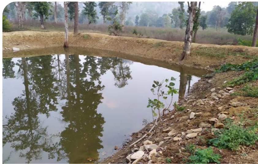
A completed water harvesting structure in Bodia, Chhattisgarh
